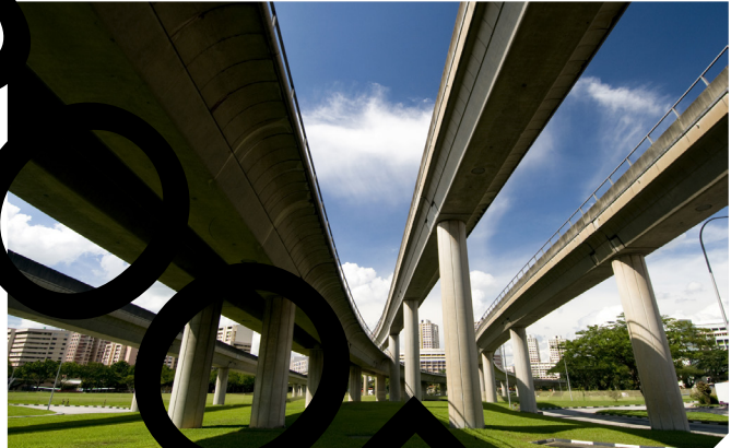
Infrastructure monitoring: vehicle and passenger detection; lighting and video surveillance control.
