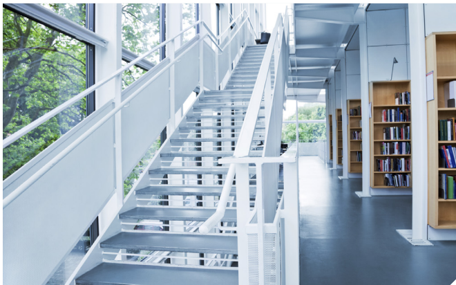
Smart building: temperature, humidity, PIR, CO 2 , and vibration detection; lighting, ventilation, and alarm control.
